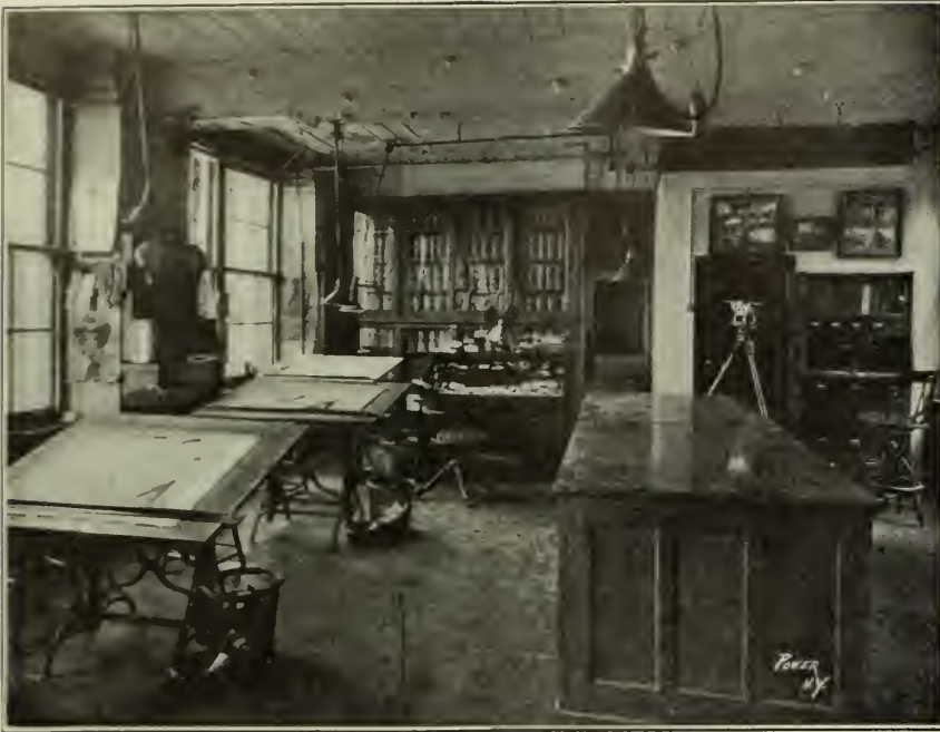
CHIEF ENGINEER'S OFFICE
